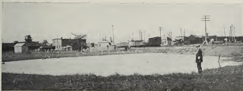
FIG. 30.—Pond caused by subsidence at Westville, Vermilion County, where 6 feet of coal was removed by room-and-pillar mining at a depth of 210 feet. Levels at surface show maximum depth of sag to be 4.7 feet. (Photo by R. Y. Williams.)
